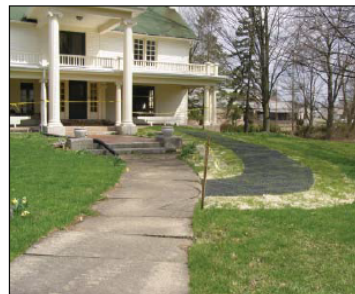
Grass pavers create a ramp without concrete and without altering the historic entrance to the building.
