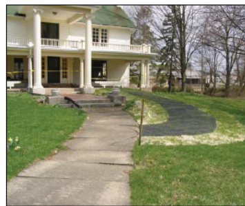
Grass pavers create a ramp without concrete and without altering the historic entrance to the building.
