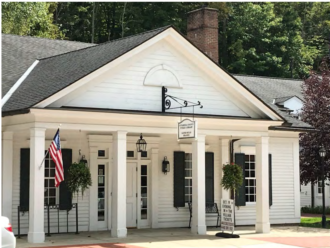
Cuyahoga County Public Library in Village Center along Chagrin River Road. CT Consultants.
